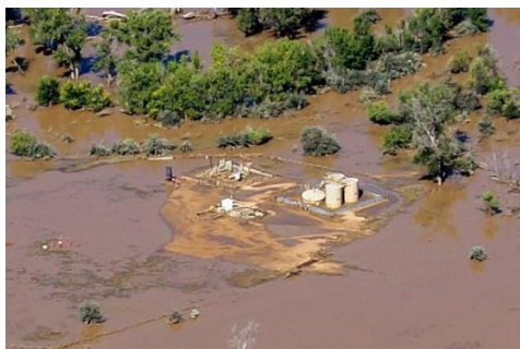
2013, Weld County Colorado. Floods inundated hundreds of fracking wells causing contamination. Source: The Aspen Times 2013
