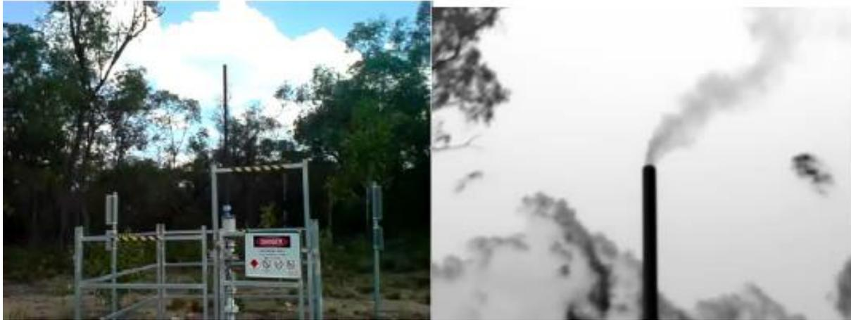
Visual and infrared images of continuous methane venting in the Queensland coal seam gas fields.
