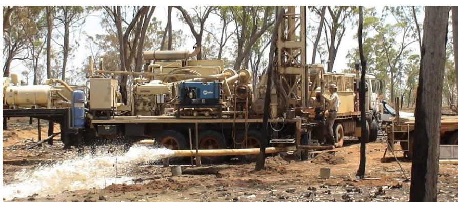
Plate 6.7 Airlifting 25L/s at RN35920
