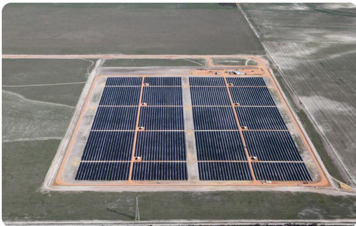
Figure 4. - Greenough River Solar Farm (Mid West WA) – 50 hectares/10 MW 71
