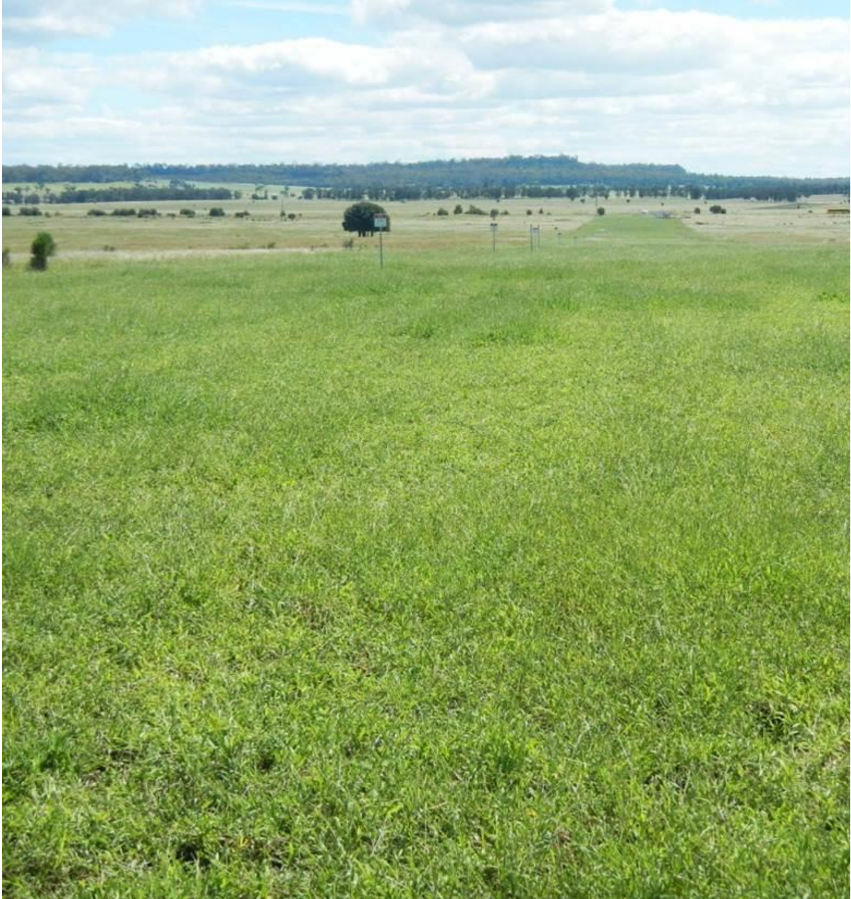
Figure 9.– Rehabilitated 48-inch gas pipeline corridor in Queensland leading to LNG plant (carries equivalent to 40,000,000 tonnes per annum of coal which would need to be transported via railway line).
