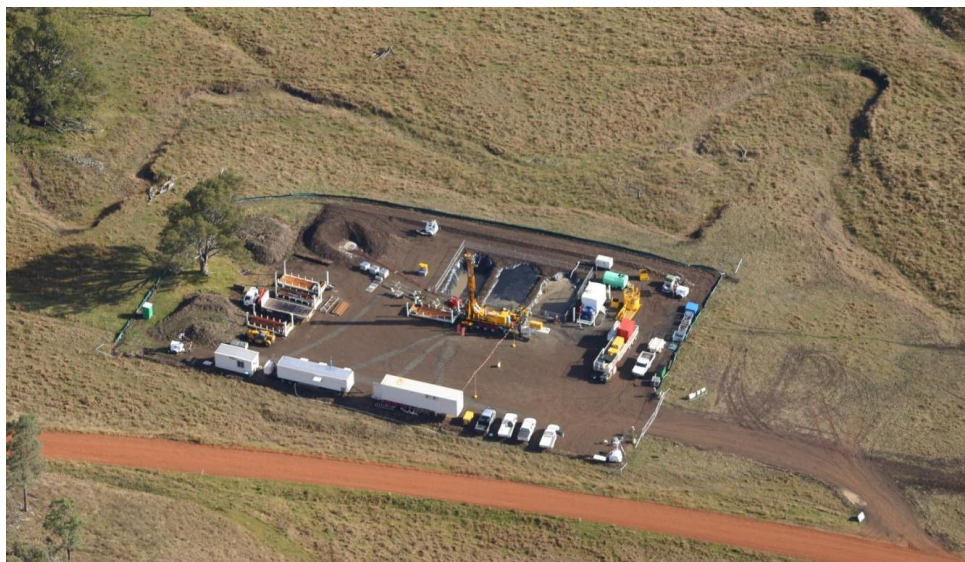
Figure 8.— Well site at Brawboy, Gunnedah Basin, NSW
