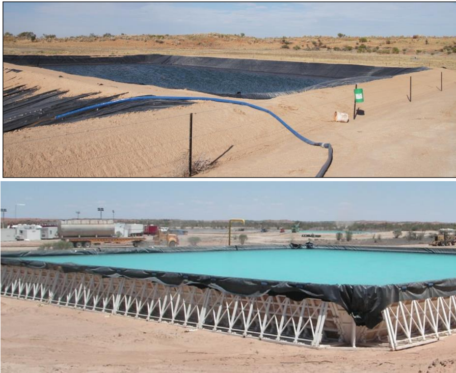
Plate 2: Examples of temporary water holding ponds used in the Cooper Basin
