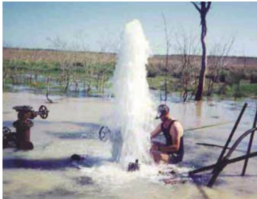
Figure 12 Example of a headwork for a flowing bore, where water supply is out of control (© Copyright, NDULC 2012).
