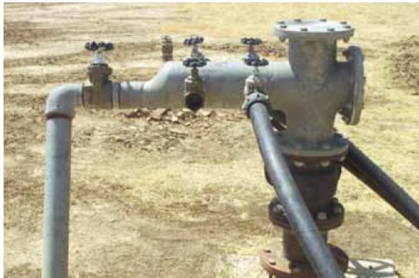
Figure 11 Example of a headwork for a flowing bore, where water supply is under control (© Copyright, NDULC 2012).
