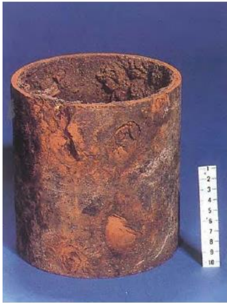
Figure 4 Examples of corrosion of bore casing (© Copyright, McLauchlan 2002).
