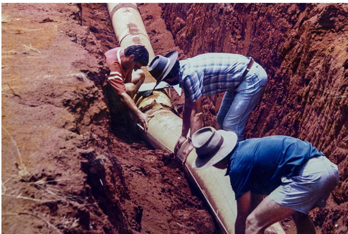
A gas pipeline is repaired after the 1988 Tennant Creek earthquake. Photo: Geoscience Australia in ABC News article: http://www.abc.net.au/news/2016-05-12/northern-territory-1988-quake-now-rated-australias-biggest/7406988
