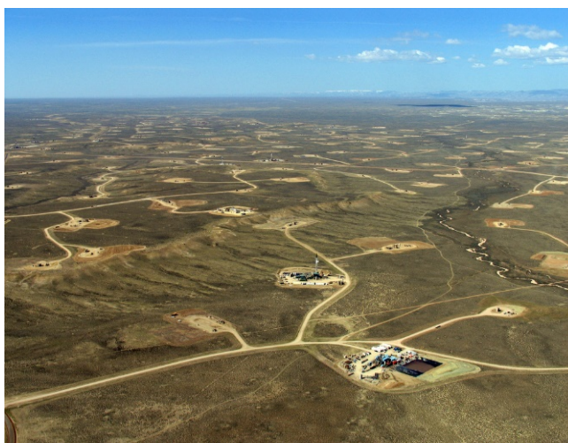
Figure 6. Well pads, access roads, pipeline corridors and other fracking infrastructure in Green River Valley, Wyoming, USA. Source: Hoffman 2012.
