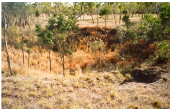
Plate 2 Sinkhole on Avago Station
