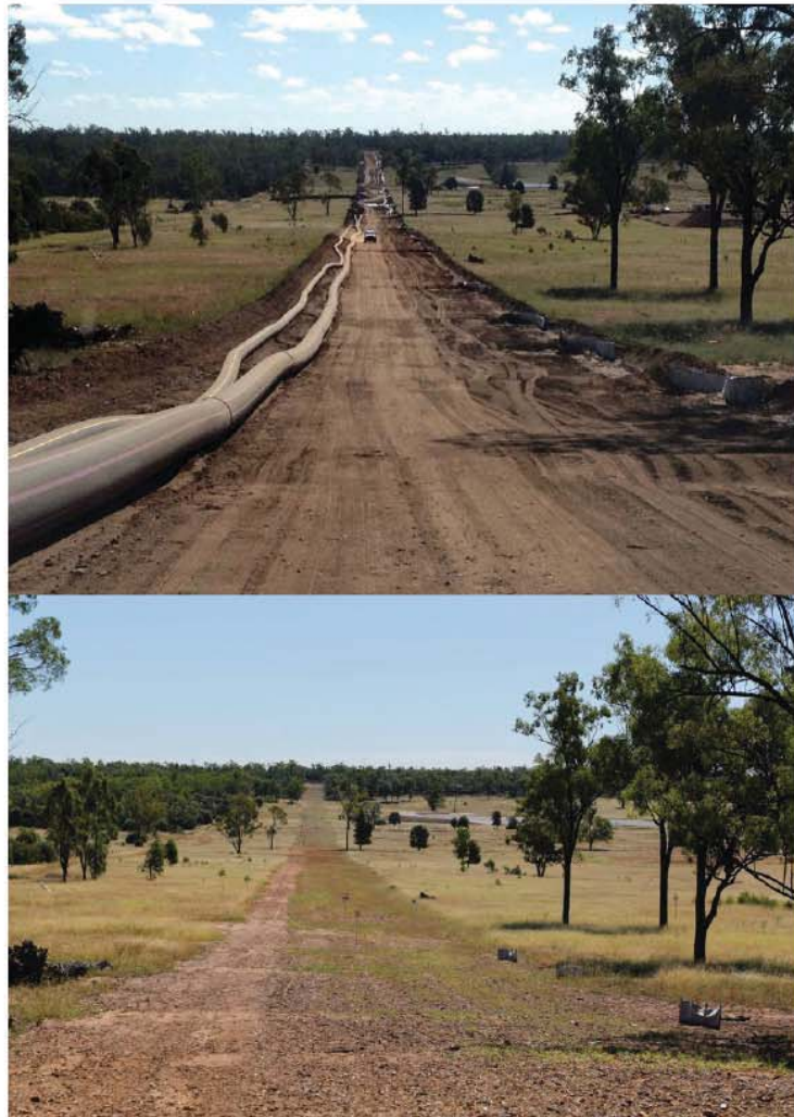
Figure 39. Pipeline during construction and following rehabilitation.
