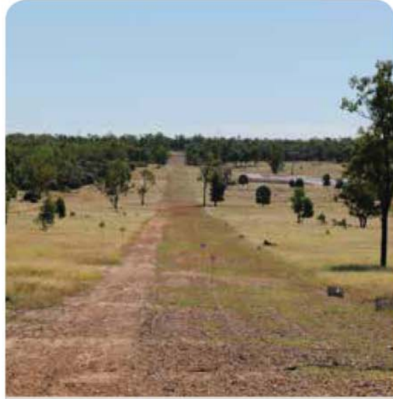
Pipeline – under rehabilitation
