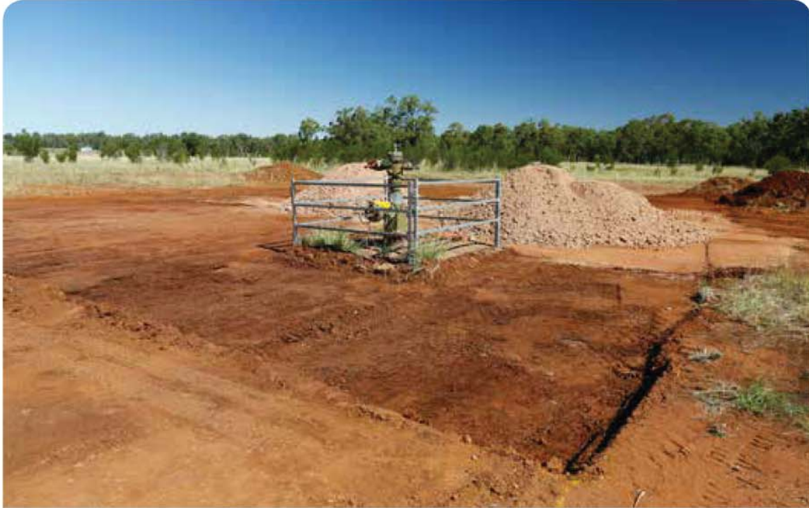
Completed CSG well; prior to installation of surface equipment
