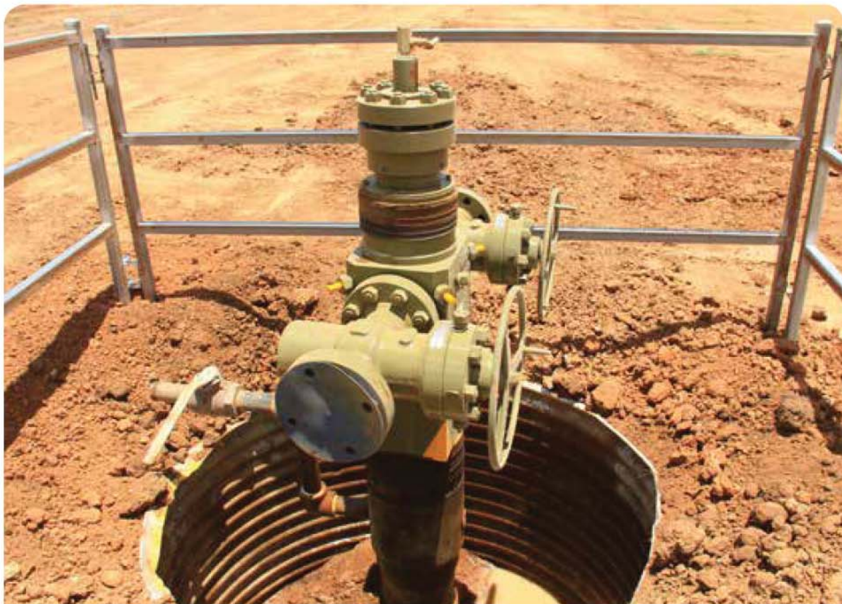
Exploration well cased and suspended prior to rehabilitation.
