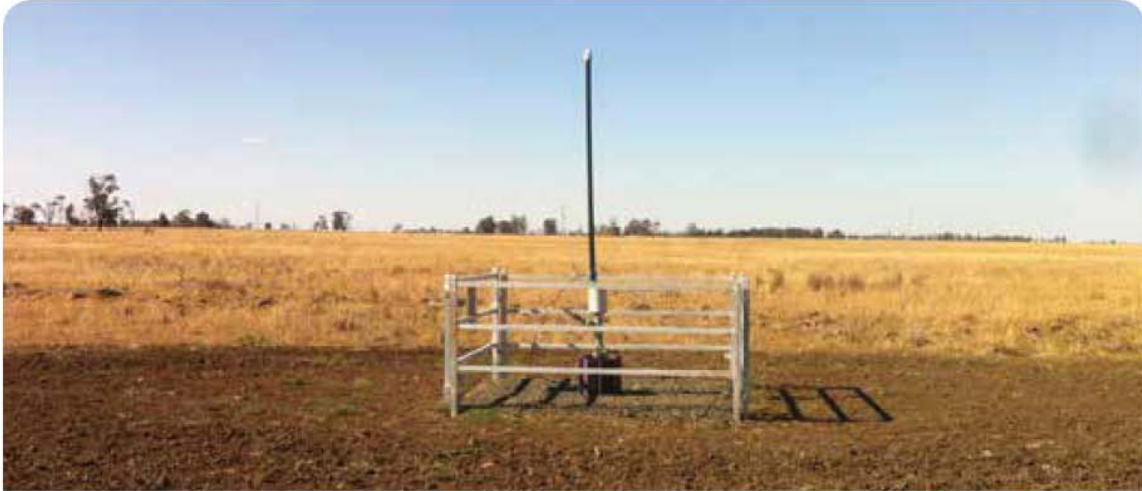
High point vent
