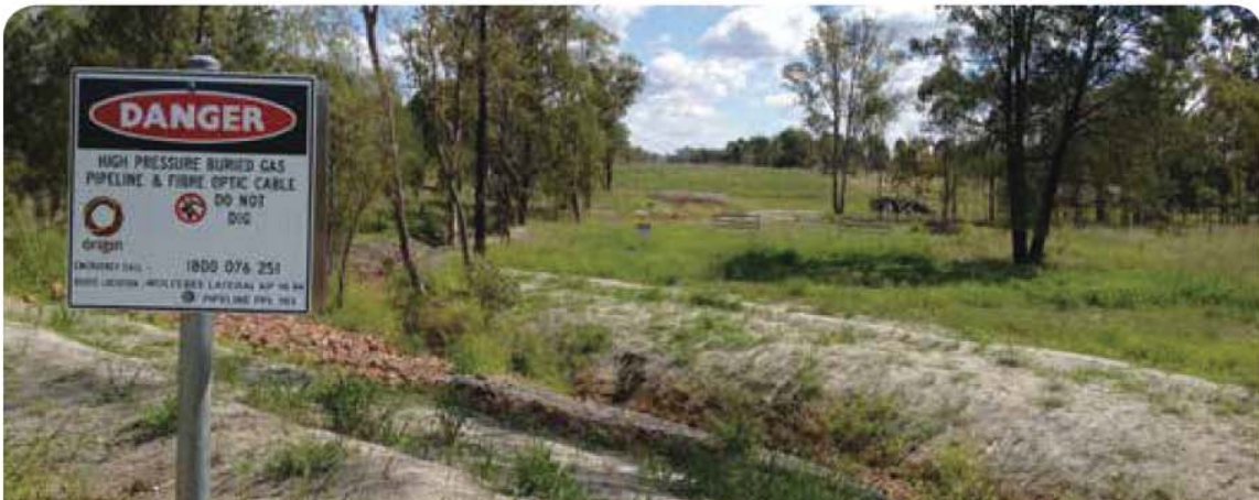
Above ground signage used along gathering and transmission pipelines
