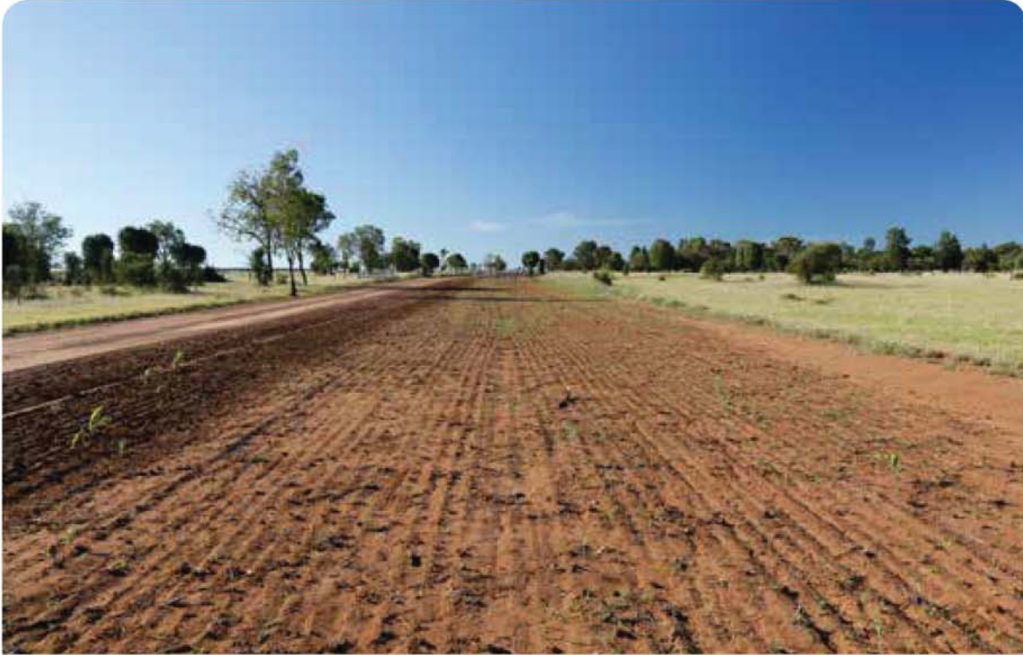
Right of Way rehabilitation at three to four weeks
