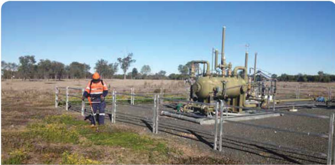
General maintenance around well
