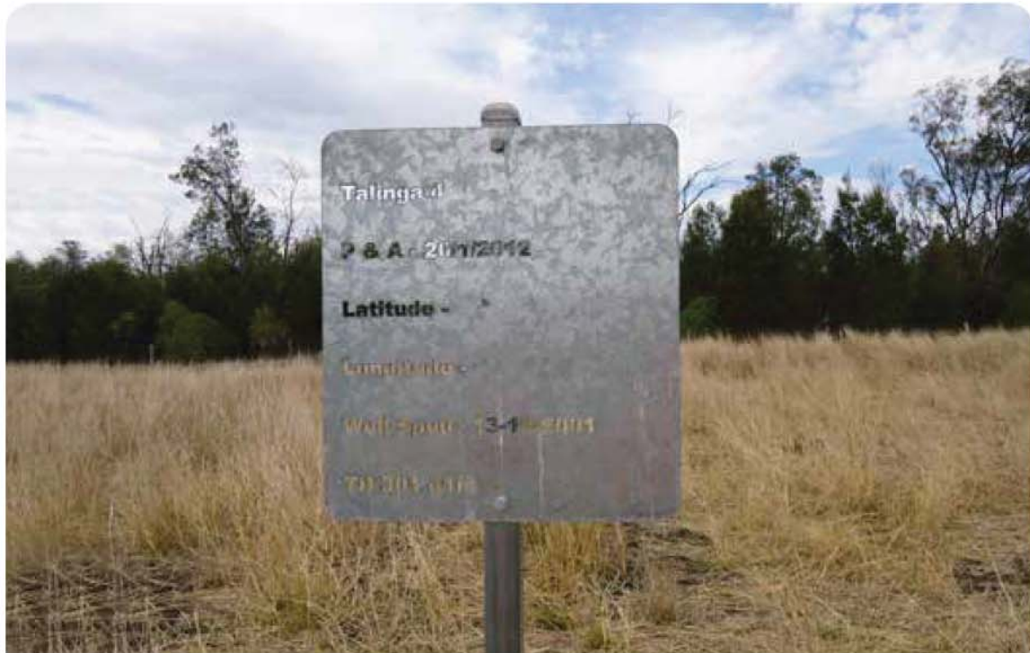
Steel marker sign for a plugged and abandoned well
