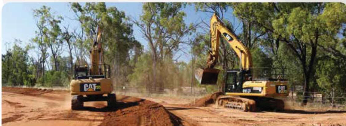
Pipeline Right of Way
