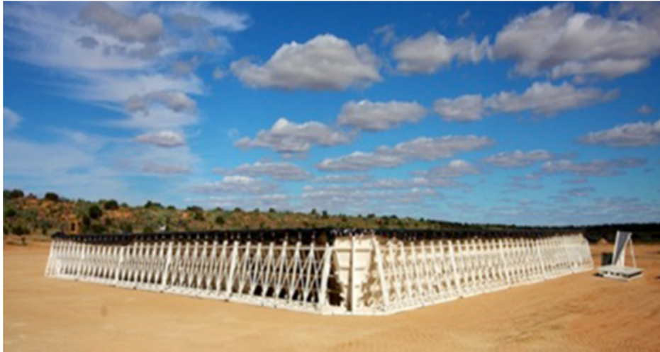
Figure 10 Above ground storage ponds used for stimulation make-up water storage and flowback water storage in the Cooper Basin. Source: Santos 2013
