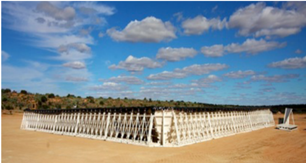
Figure 43 Above ground storage pond used for stimulation make-up water storage and flow back water storage in the Cooper Basin. Source: Santos, 2013.
