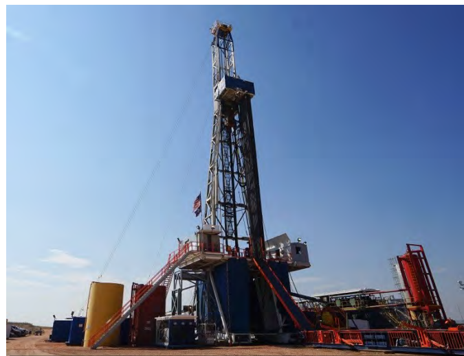
Chesapeake drilling rig employing horizontal drilling techniques
