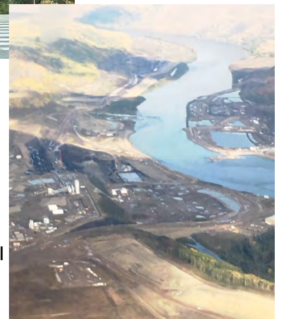
The dam being constructed at Site C.
