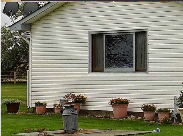
The water well that Louis said was affected by poor gas well construction
