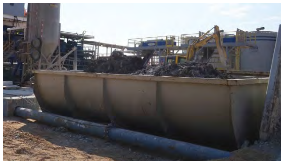
Drilling muds being loaded into skip bin
