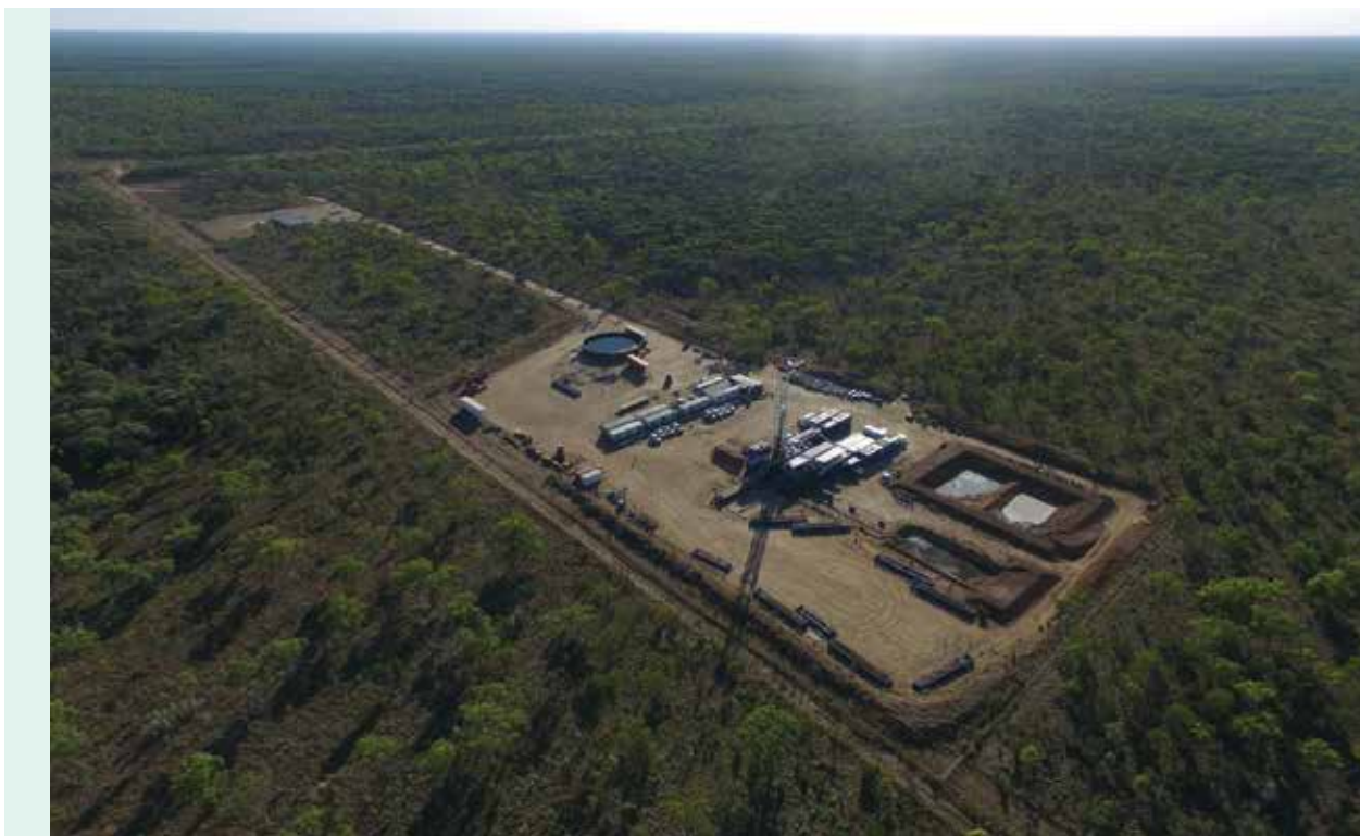
Amungee NW-1H wellsite in EP98 during drilling operations (30-60 days): Source Origin.
