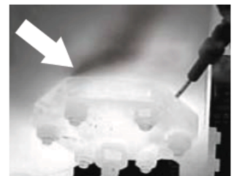
The sniffer is detecting gas but is unable to trace its source, whereas this thermal image shows the leak source clearly on the left.
