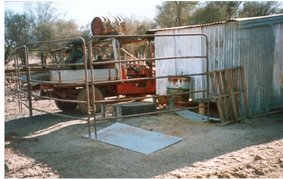
Plate 4 - 'Bulwaddy bore' at Avago Station
