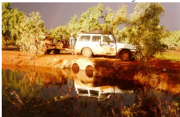
Plate 7 - Birdum Creek at Western Creek Road culvert (April, 2000)
