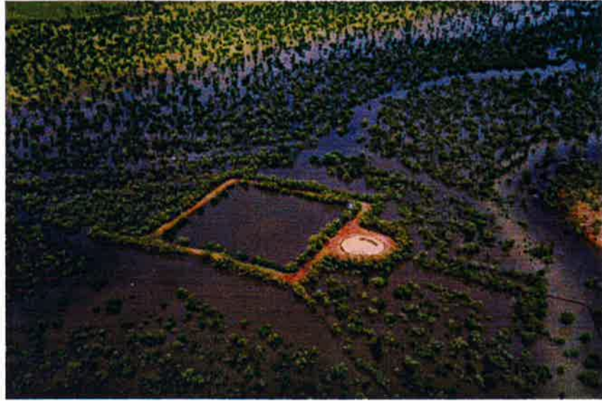
Plate 9 Cedar Lagoon Tank, Auvergne, an off-stream excavated tank with above ground storage, note the turkey nest on the right edge of the tank, used to gravity feed water to the troughs.
