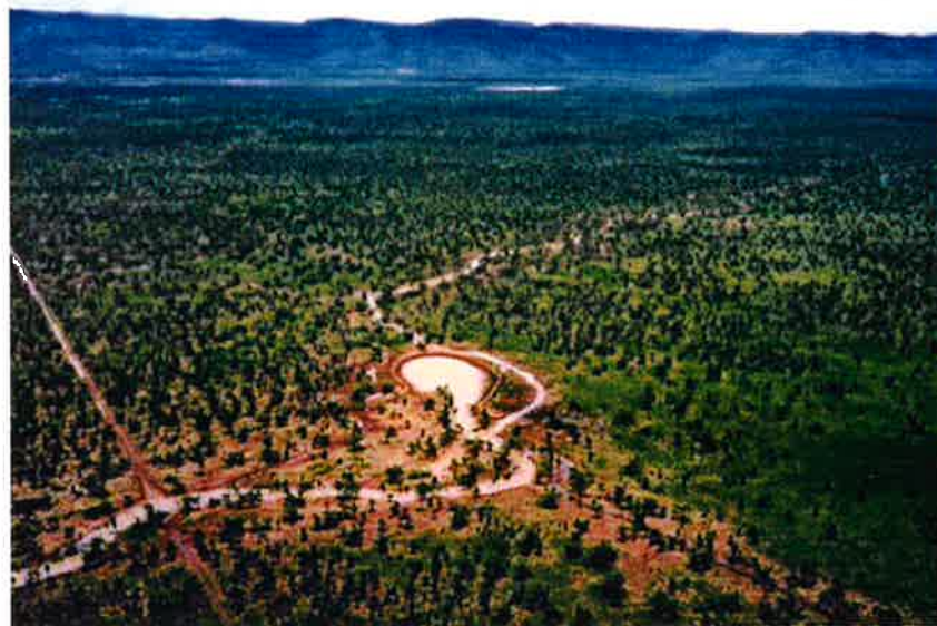
Plate 8 Horseshoe Dam, Auvergne, an off-stream excavated tank with a short inlet channel.
