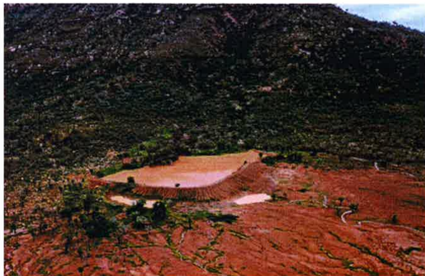
Plate 10 Burkes Dam, Bradshaw, a hillside storage.
