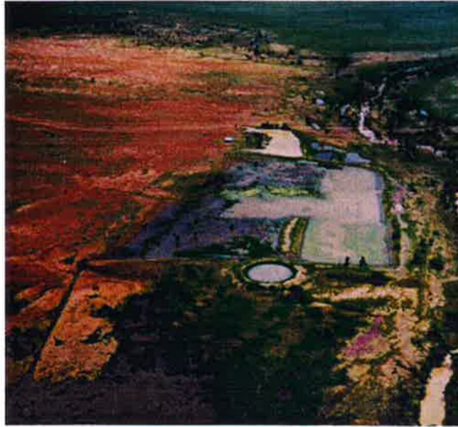
Plate 11 Police Hole Tank, Auvergne, a drainage line tank.
