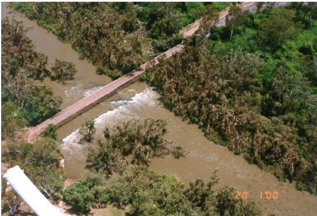
Photo B1 Katherine River at Low Level Crossing
