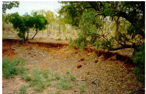
Plate 4 Sinkhole at Hidden Valley Station
