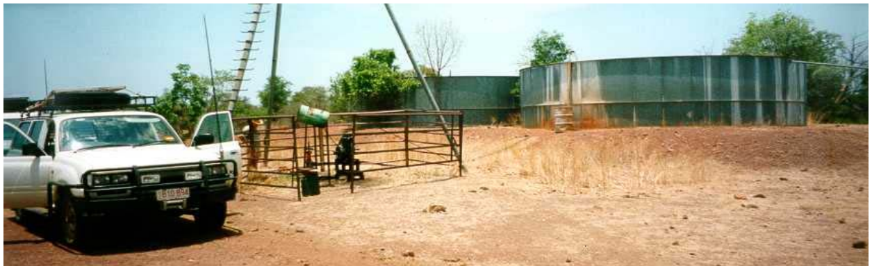
Plate 19 'D' bore and ground tanks at Kalala Station
