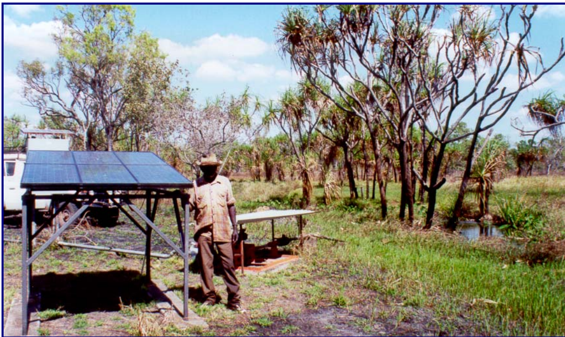
Plate 2 Hitler at the Mount Catt Water Supply. The Pump is Run by Solar Energy.
