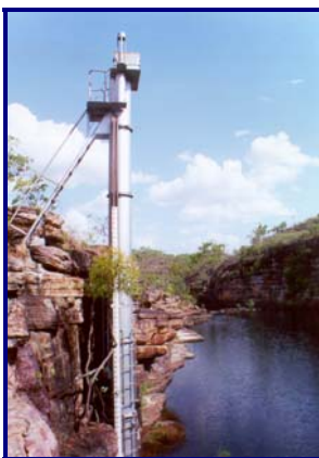
Plate 4 Gauging Station at Liverpool River GS 8230237
