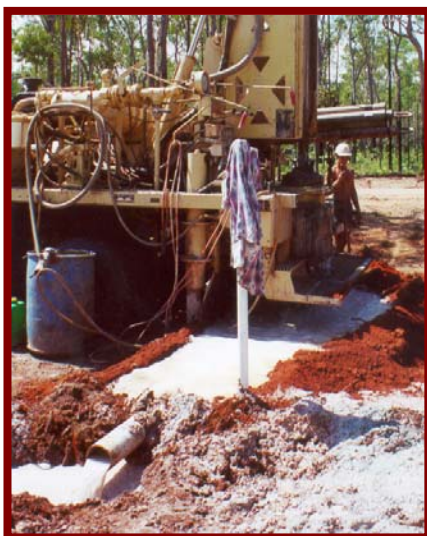
Plate 14 Airlifting 10 l/s at the bore near Jungle Creek
