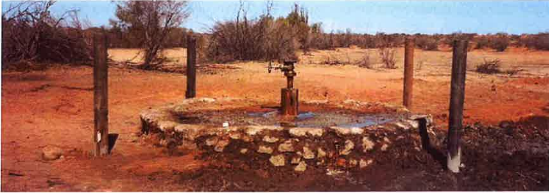
Pic: Anacoora Bore Construction June 2000
