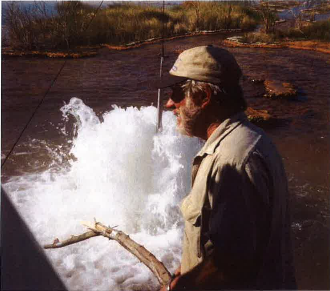
Pic: McDills – attempting to lower logging tool into uncontrolled bore
