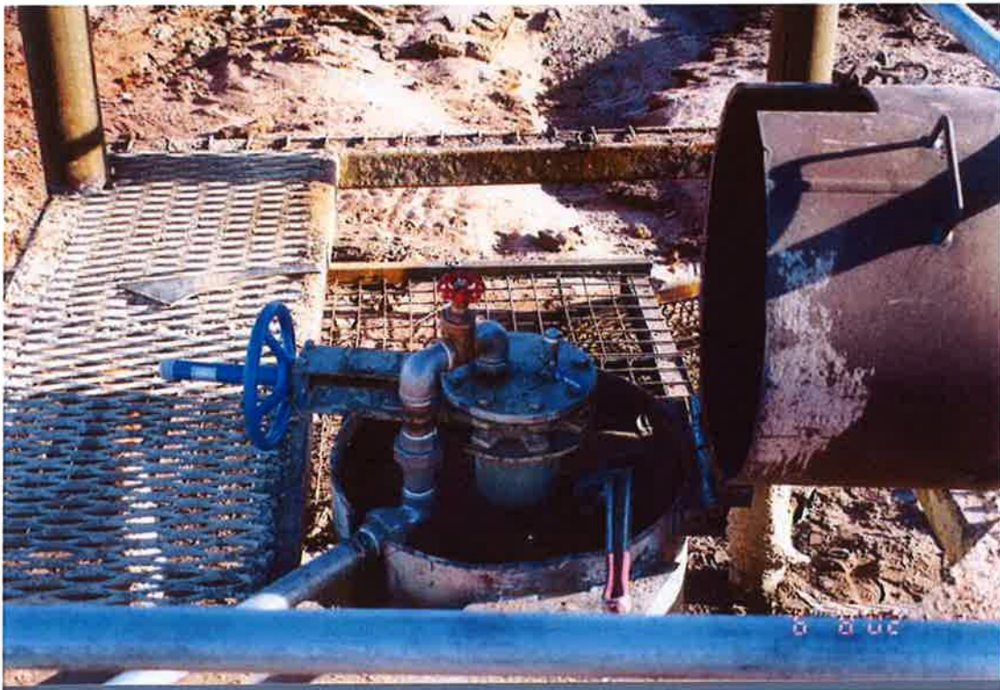
Pic: McDills headworks after rehabilitation
