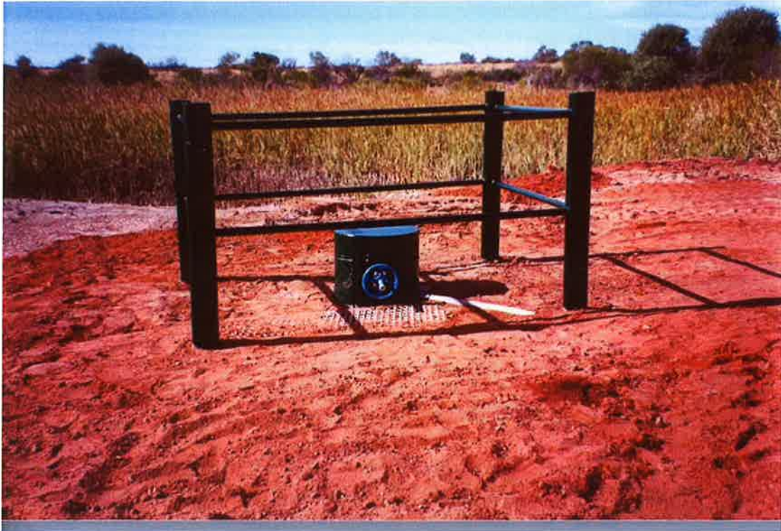
Pic: McDills headworks after rehabilitation
