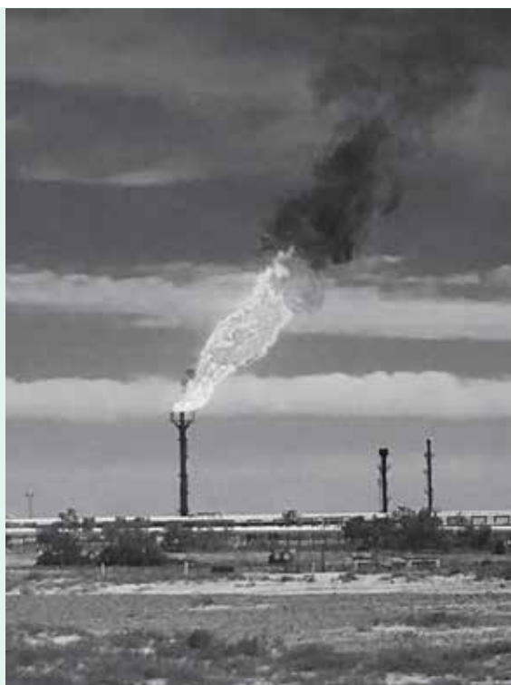
Flaring at a gas processing facility in Australia.
