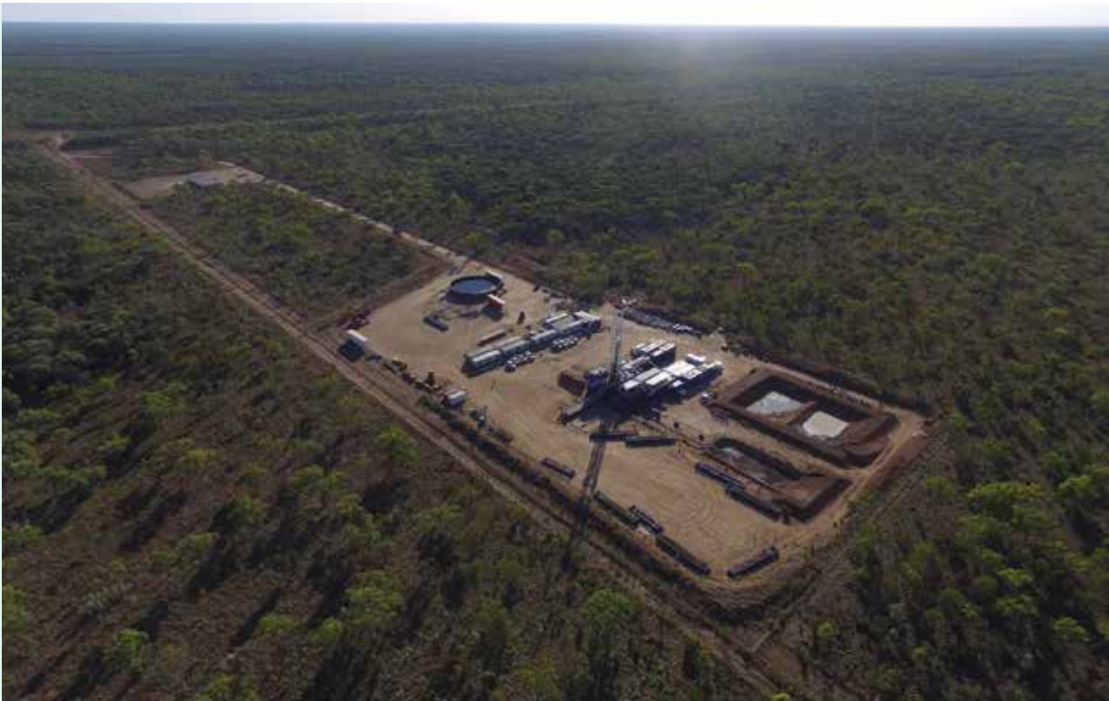
Amungee NW-1H wellsite in EP98 during drilling operations (30-60 days): Source Origin.
