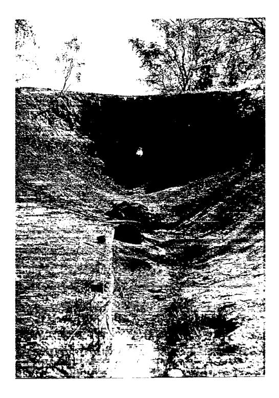
Plate 1: Saddle Creek Dam, showing damage to the inlet pipe and erosion of the bund at the inlet
